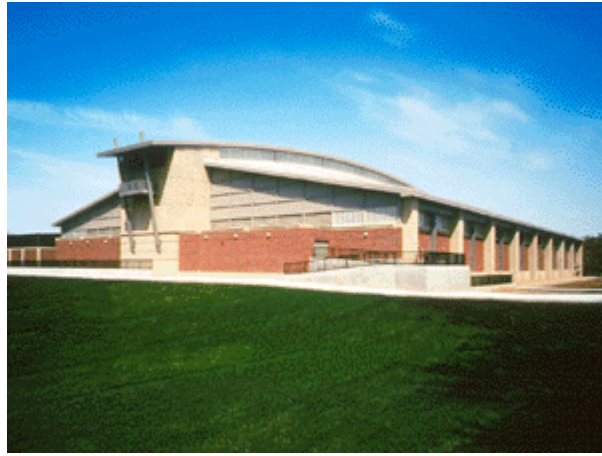
The Indoor Football Practice Facility at The University of Illinois at Urbana/Champaign Champaign, Illinois Tylk Gustafson Reckers Wilson Andrews, LLC.
