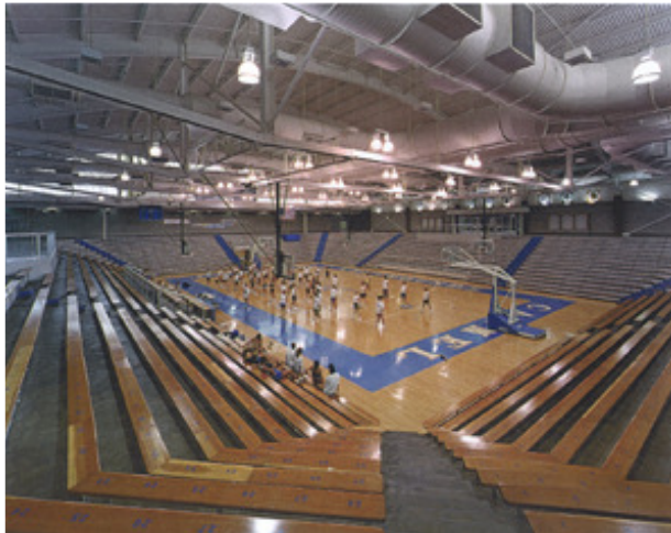
Carmel High School Basketball Arena Roof Replacement Carmel, Indiana OWP&P
