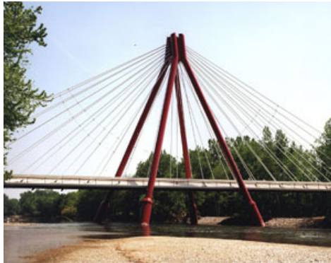
East Fork Cable-Stayed Bridge Columbus, Indiana J. Muller International
