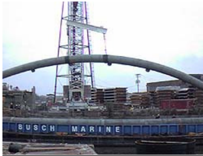
Damen Avenue Bridge J. Muller International
