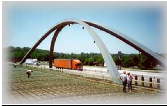
Columbus Gateway Arch Bridge
